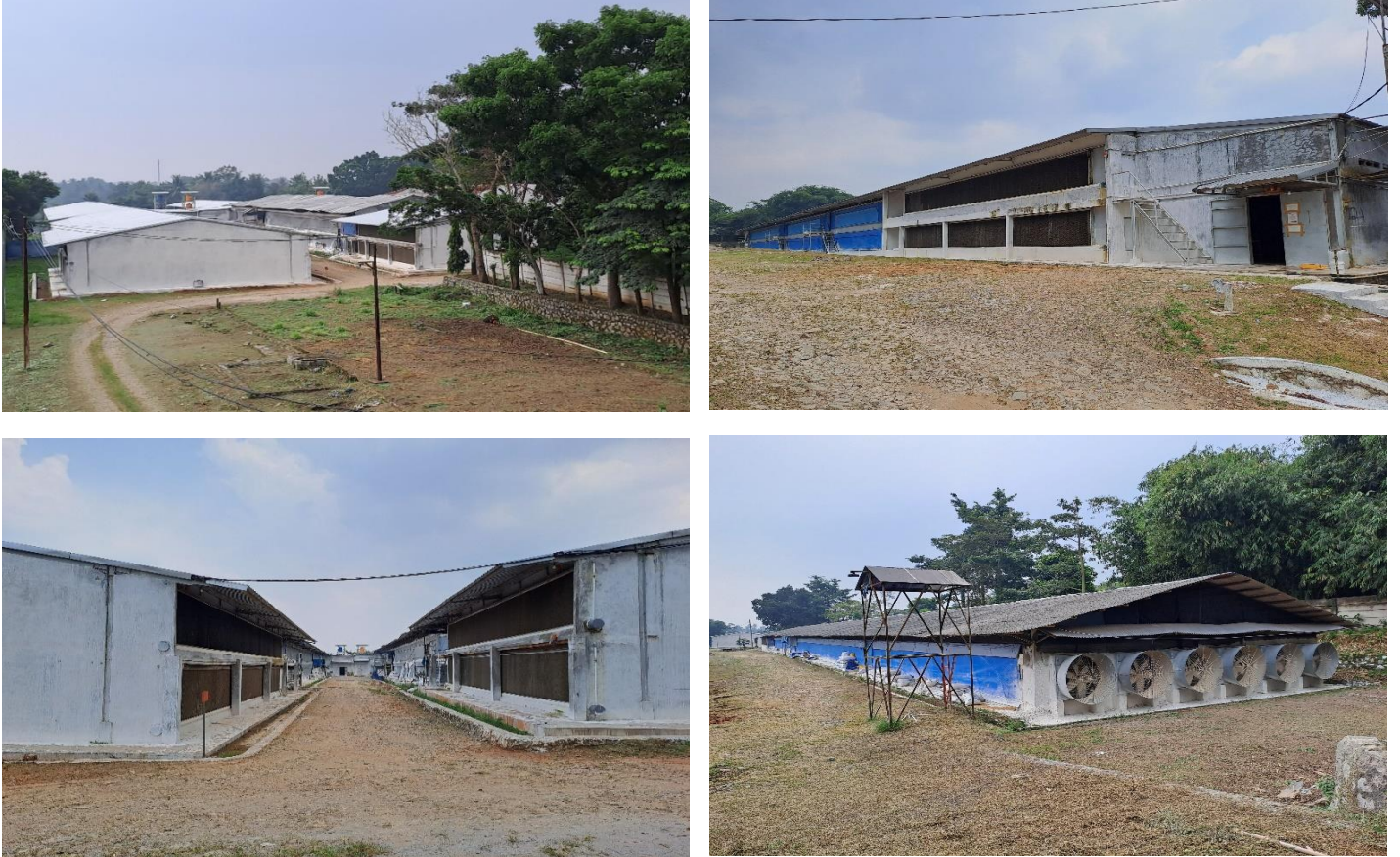
Figure 12: Cisoka commercial farm – 4.6 ha land area contains four double- and one single-deck barn closed house system
