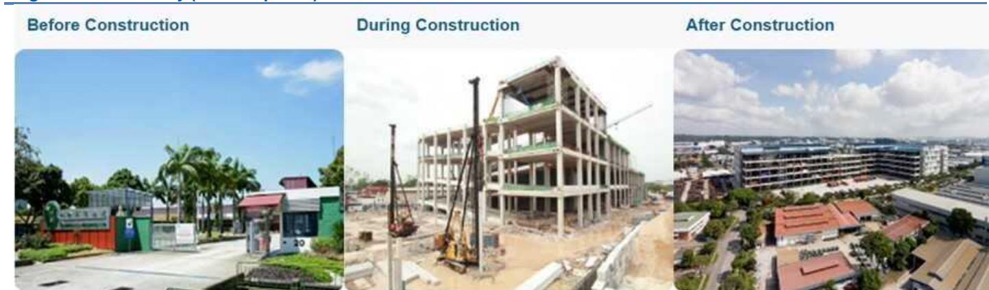
Figure 12: 20 Gul Way (redevelopment)
