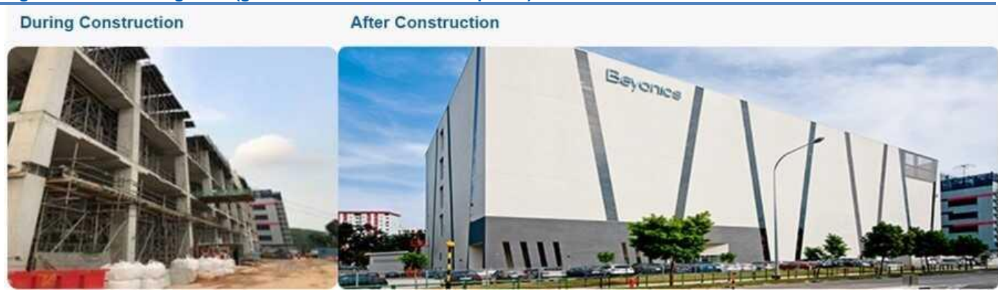
Figure 13: 51 Marsiling Road (greenfield build-to-suit development)
