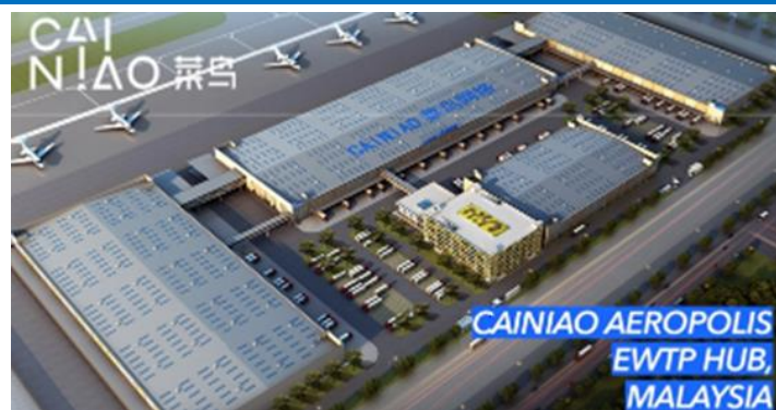
Figure 45: Aerial view of Cainiao Aeropolis eWTP's future development
