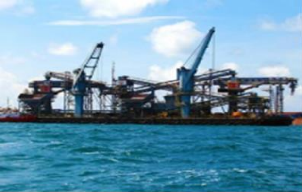
Figure 30: Floating loading facility
