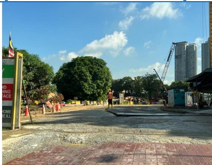
Figure 1: Construction site of RTS station in Bukit Chagar
