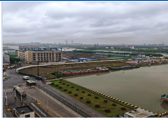
Figure 17: Wharf in front of Hangzhou Food Park
