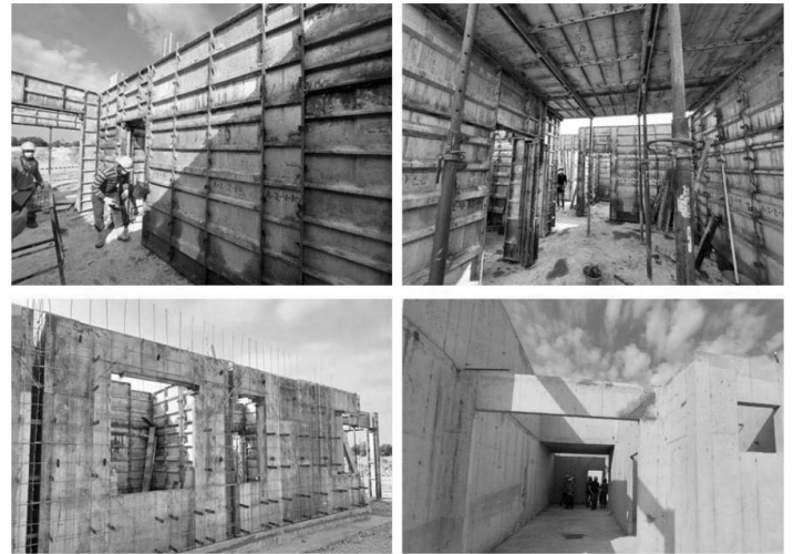
Figure 13: Aluminium formworks systems at sites
