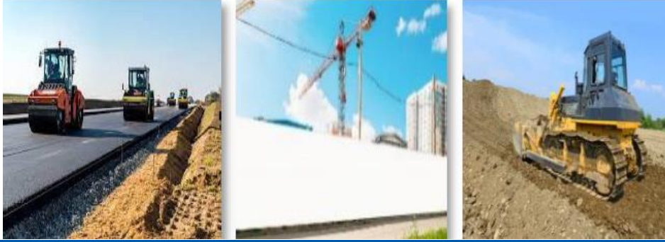
Figure 20: Examples of other related services – roadwork, hoarding work and earthwork
