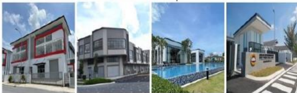
Figure 19: Examples of non-residential buildings – industrial, commercial, purpose-built and institutional
