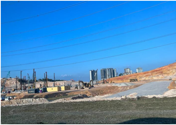
Figure 1: Land levelling works for TM Nxera DC in Iskandar Puteri are mostly done
