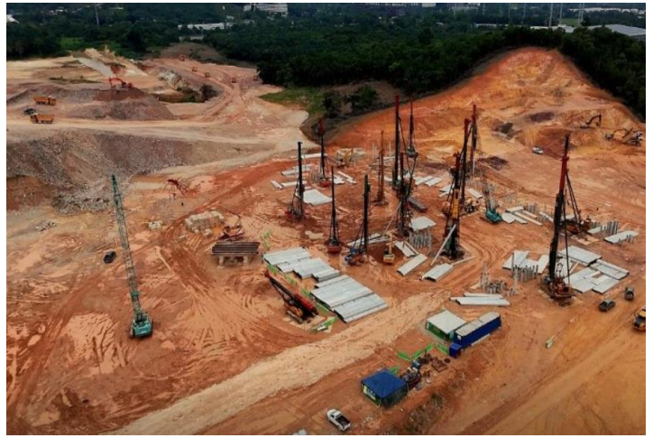
Figure 2: Aerial shot of piling works for TM Nxera DC (picture taken in May 2025)
