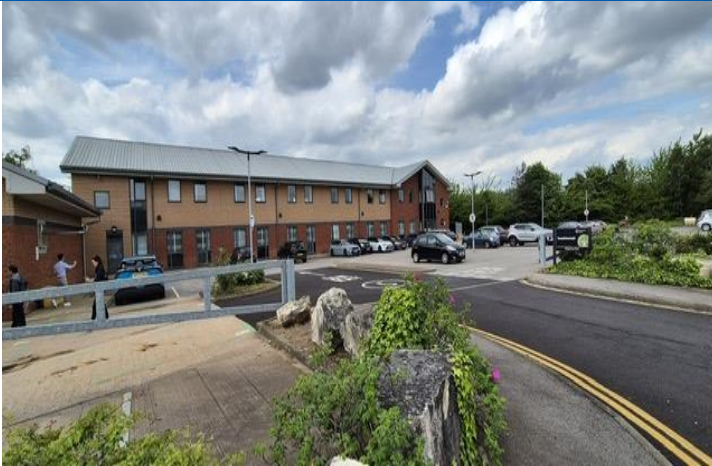
Figure 32: Bradmarsh Business Park
