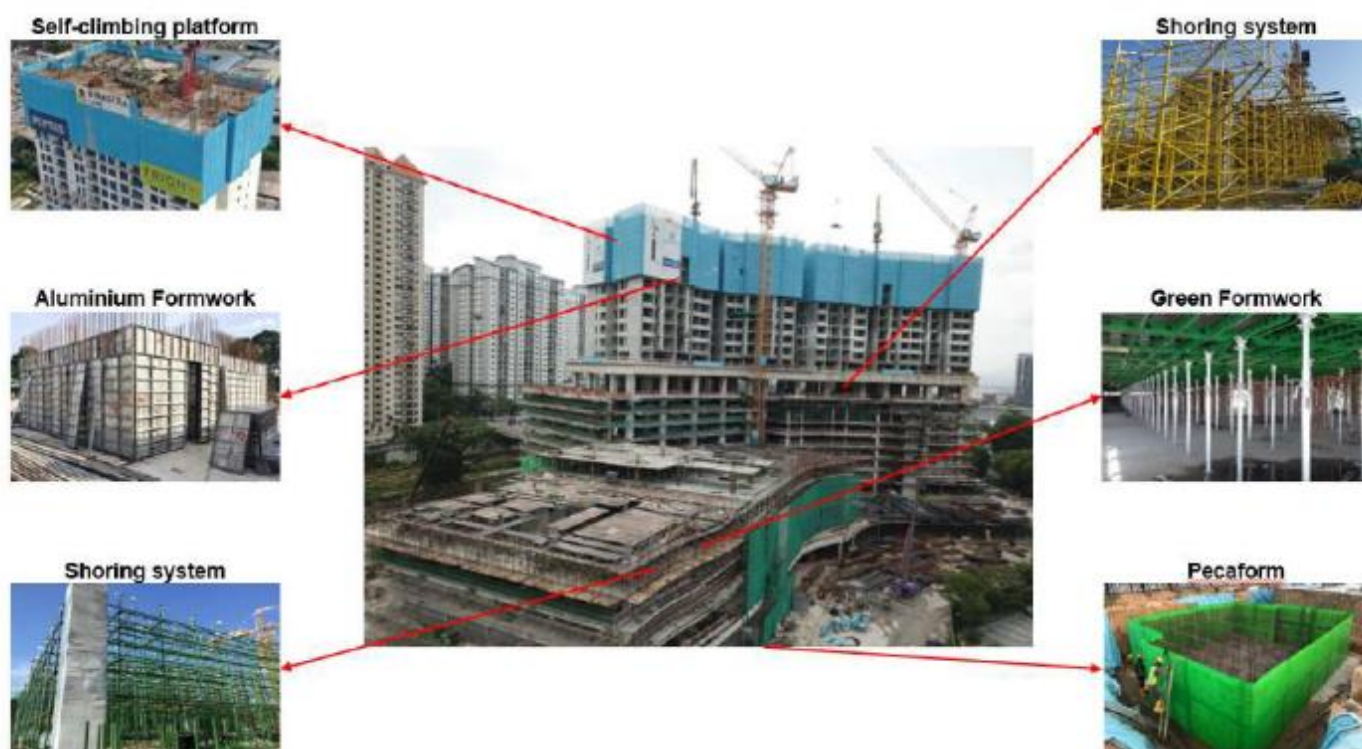
Figure 11: Example of CME Solutions used in different segments of a high-rise building
