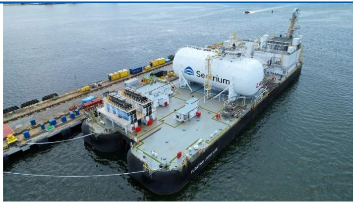
Figure 10: The first stacked ESS in South-East Asia
