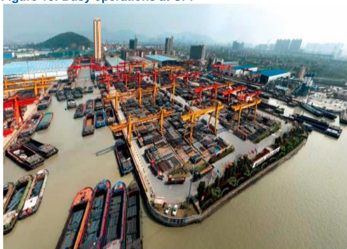
Figure 16: Busy operations at CPI
