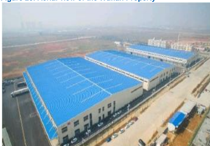
Figure 26: Aerial view of the Wuhan Property
