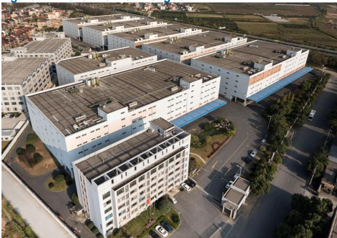
Figure 14: Aerial view of Hengde
