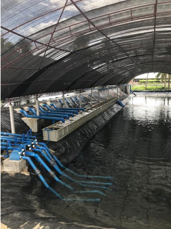
Figure 5: Treated seawater reservoir
