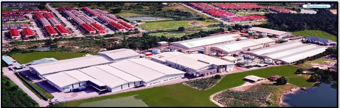
Figure 18: Rubberex’s manufacturing plant in Ipoh
