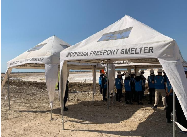
Figure 1: Freeport project in progress I
