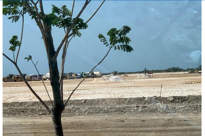
Figure 2: Freeport project in progress II
